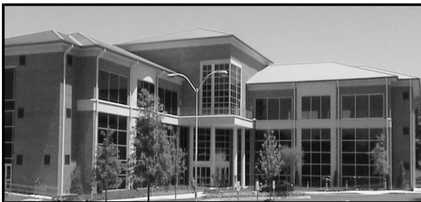
THE DIVISION IS HOUSED IN THE:
